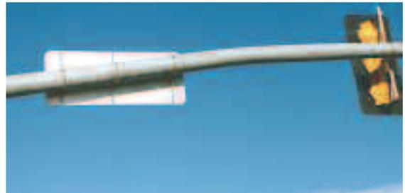
This 2' x 6' sign was assembled and installed with Medium Channel Extrusion and Universal Channel Clamps. Built for high wind loads, the sign can be quickly mounted level in spite of the mast arm angle.
