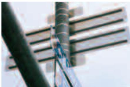
San Diego, California has been improving and enlarging their signs. SIGNFIX was chosen because of its ease of application and strength. These 10' wide, 18" tall signs were installed using Medium Channel Extrusion and Universal Channel Clamps. Installation time less than 5 minutes per sign.
