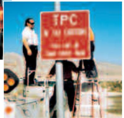
This 4' x 4' .080 gauge aluminum sign was installed in less than 5 minutes using SIGNFIX Large Corner Angle Channel Extrusion and Universal Channel Clamps. Using the SIGNFIX Channel Spacing Software, the sign was designed for a 100 mph wind load according to AASHTO specifications.
